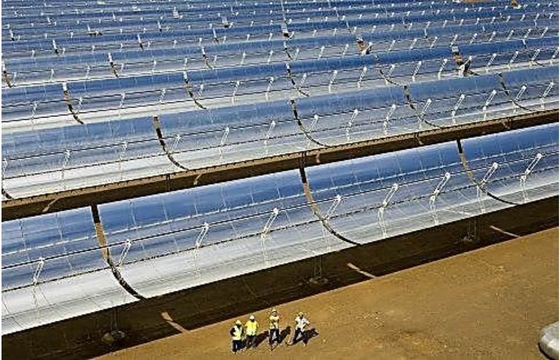
Figure (1.1): Parabolic Trough Collector [7]
