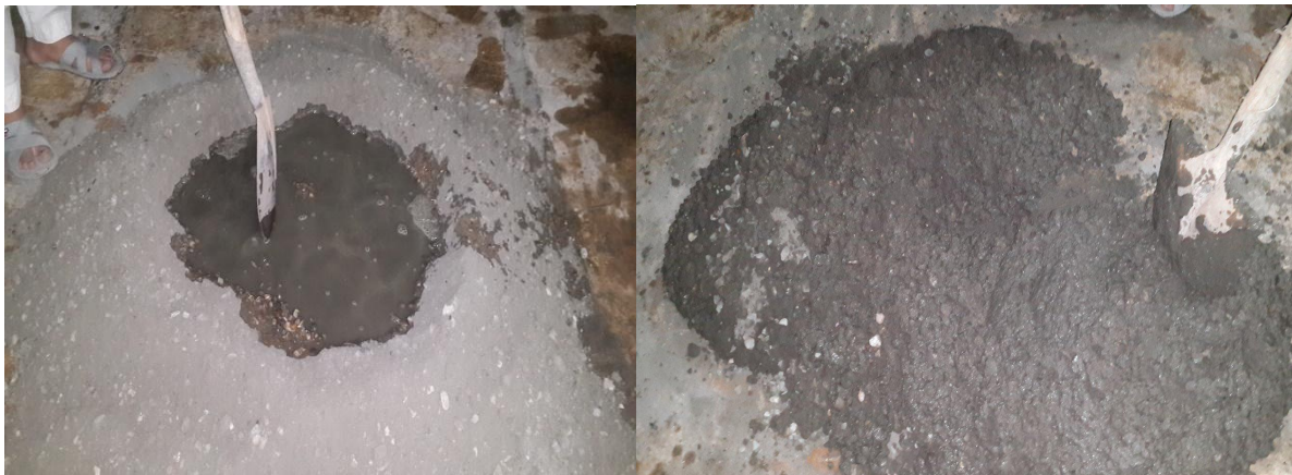
Plate (3-4): Mixing concrete
