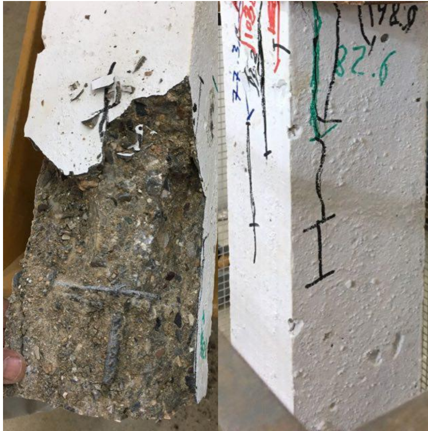
Plate (4-27): Failure Pattern for Column (HS4)
