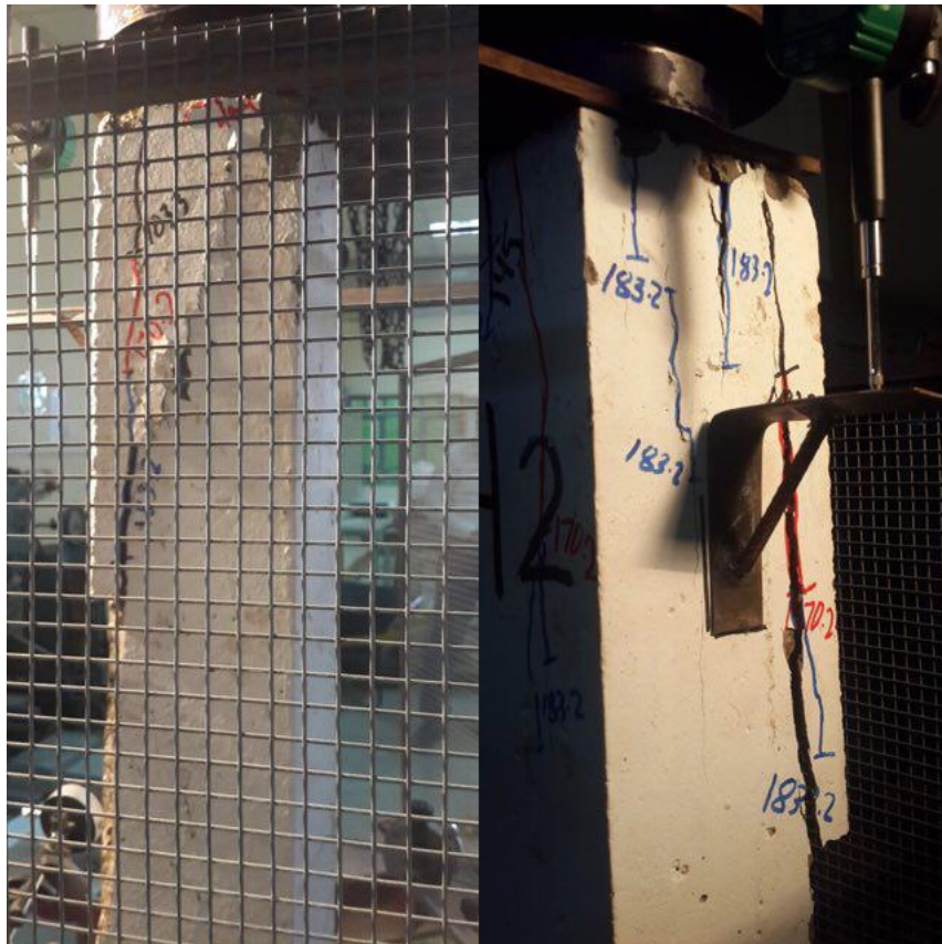
Plate (4-13): Failure Pattern for column (H2)
