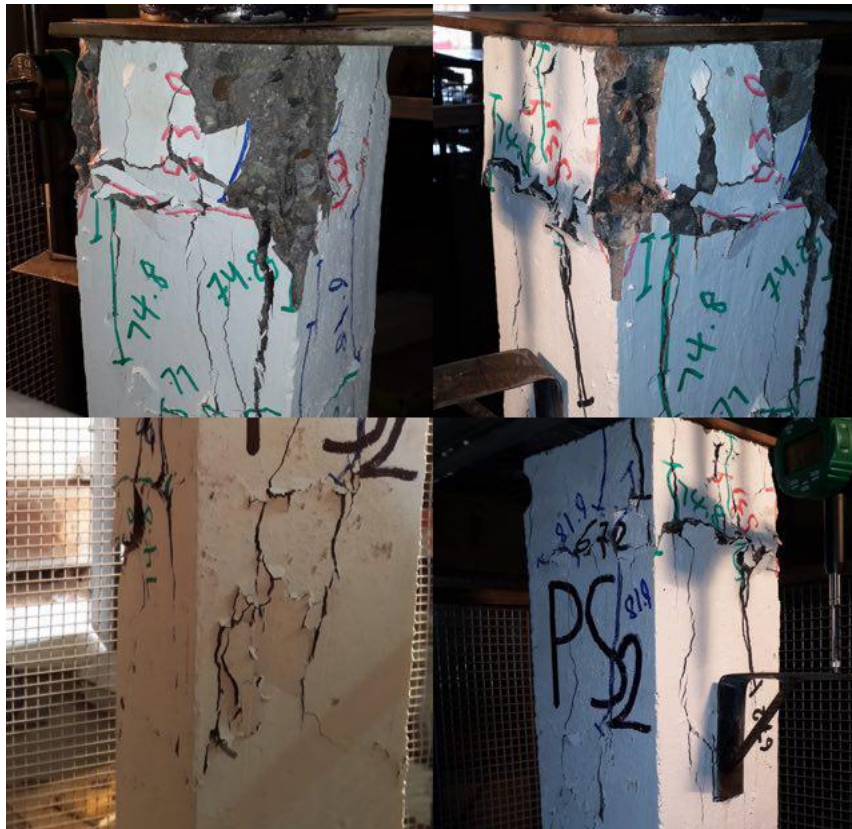
Plate (4-21): Failure Pattern for column (PS2)
