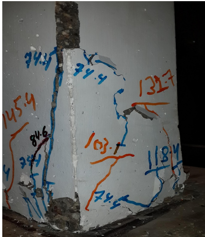
Plate (4-12): Failure Pattern for column (RS3)
