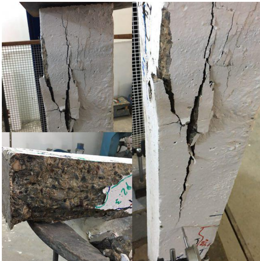
Plate (4-15): Failure Pattern for column (H4)
