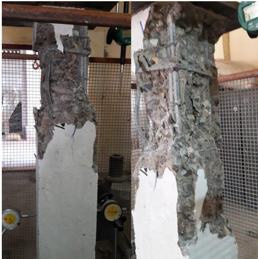
Plate (4-18): Failure Pattern for Column (NS3)
