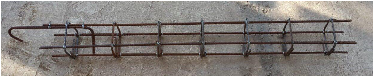
Plate (3-7): Reinforcement cage of columns
