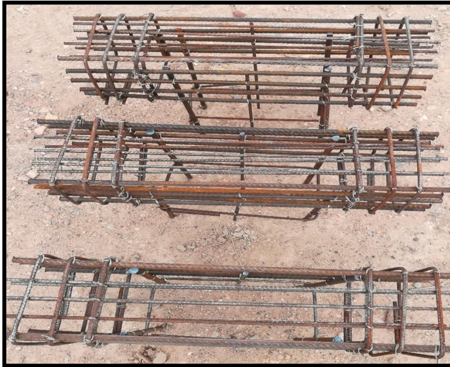
Plate 3. 6 Steel reinforcement cage of pier specimens
