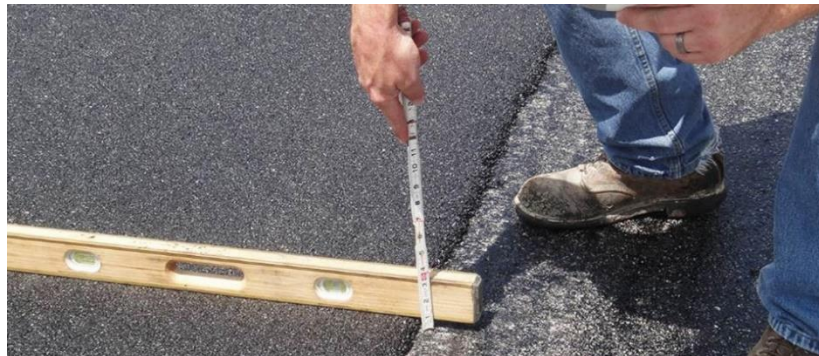
Plate 2-1 Thin Hot Mix Asphalt (HMA) Overlay ( http://fp2.org/ )
