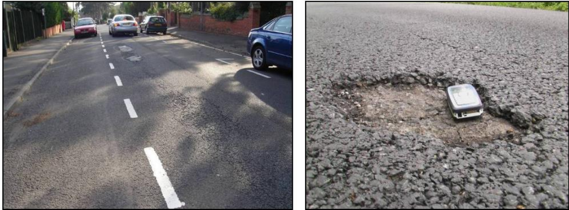
Plate 1-1 Most common problems with TAO: raveling (left) and delamination (right) (Sandberg et al., 2011)
