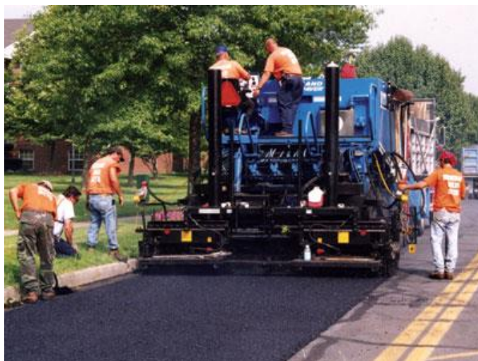
Plate 2-2 Paving Ultra-Thin Hot Mix Asphalt in Salisbury, Maryland ( http://www.ejbreneman.com/Ultra-Thin-Hot-Mix.html )
