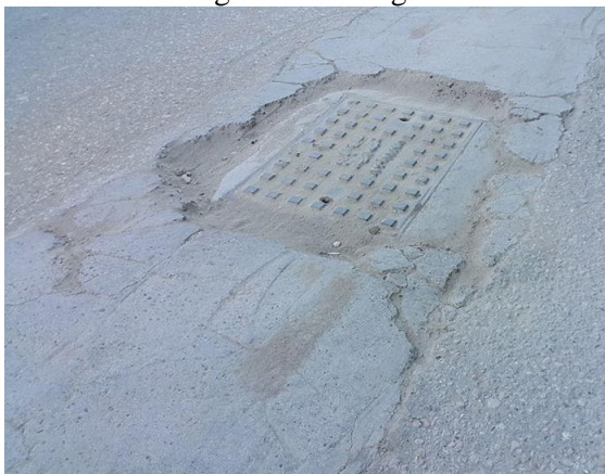
G. Utility Cut Patching
