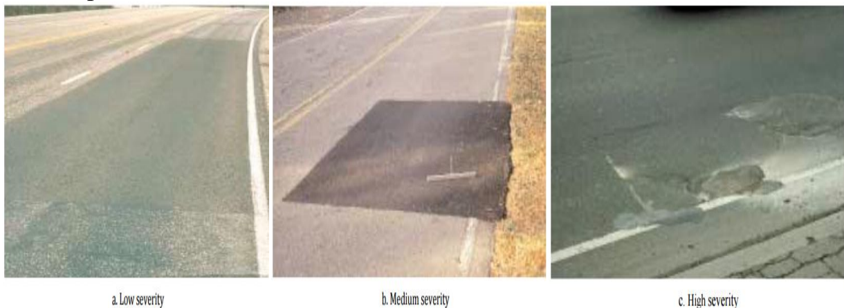
Figure (A-14) patching and Utility Cut Patching
