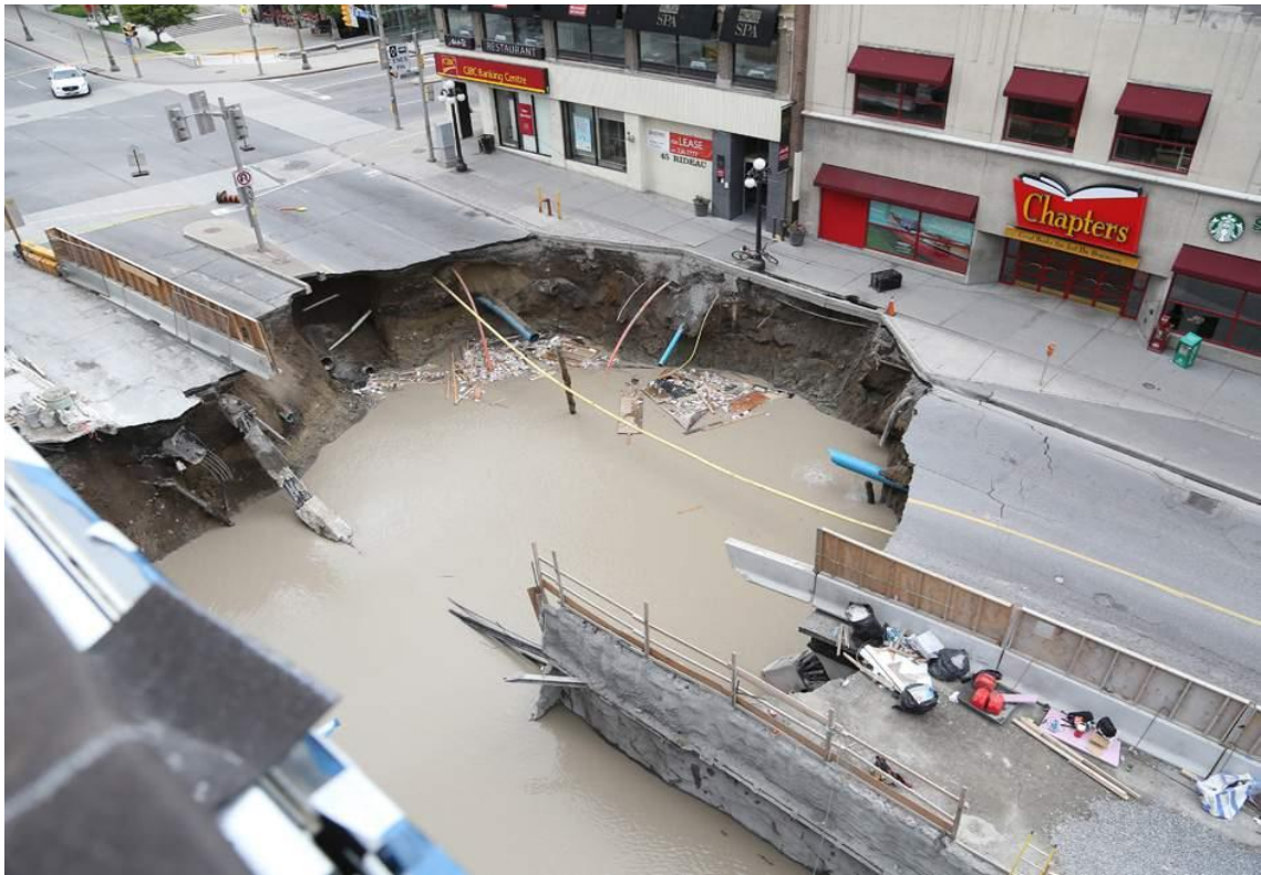
Figure 1-1 Photograph of a sinkhole accident occurred in Ottawa downtown, (BBC, 2016)
