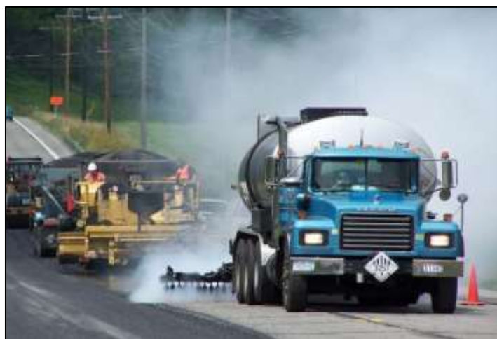
Figure 2-7 HMA paving process.
