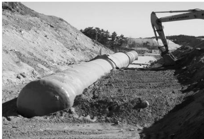
Plate (2-8): installation of pipe in site(Kim et al., 2012)
