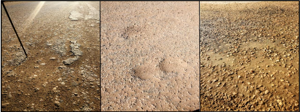
Fig. 4.39: The stripping failure in the streets that has the most flooding events in duration
