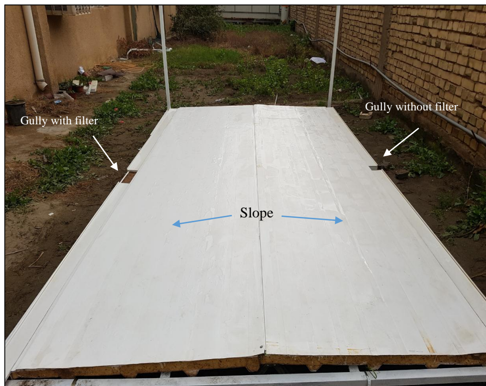
Figure (4-4) Floor slopping
