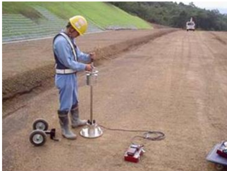
Figure 2.8 : Light weight deflectometer test device
