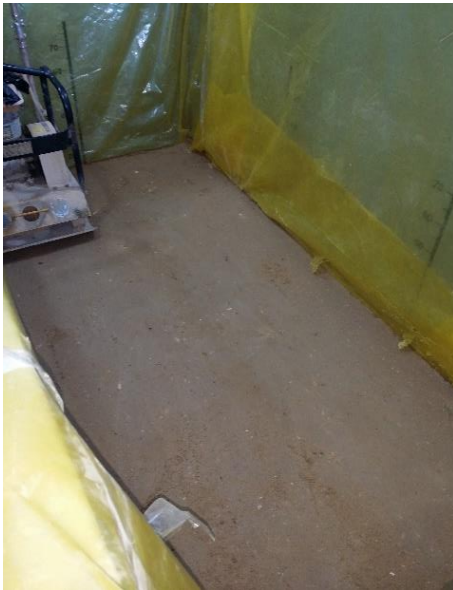
a) Compacted subgrade layers
