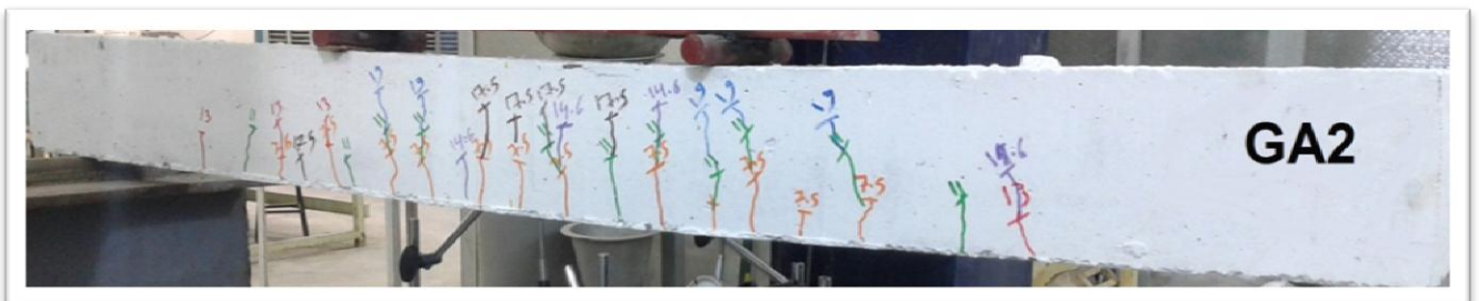
Figure (4-62): Crack patterns of beam GA2
