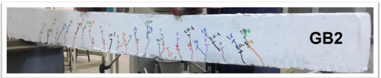
Figure (4-63): Crack patterns of beam GB2
