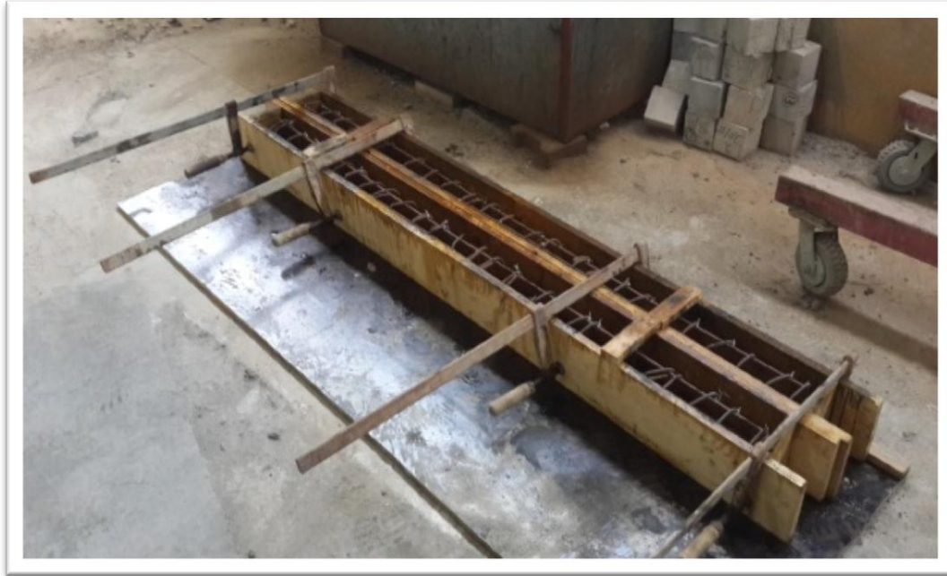
(a) Preparing the molds for casting
