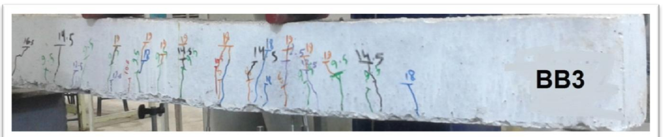
Figure (4-65): Crack patterns of beam BB3
