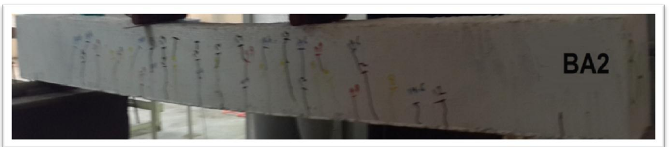
Figure (4-60): Crack patterns of beam BA2
