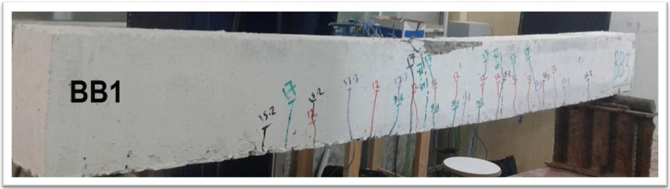
Figure (4-56): Crack patterns of beam BB1
