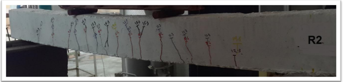
Figure (4-59): Crack patterns of beam R2
