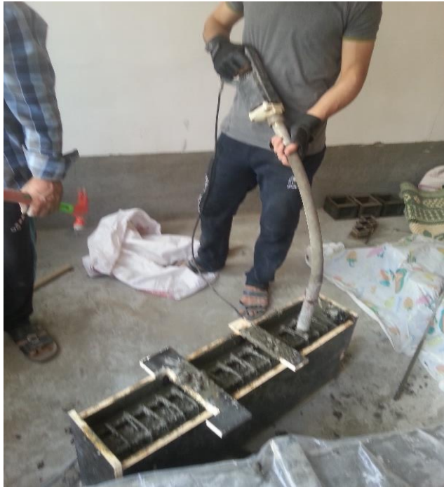
Plate (3.5) Compact the concrete using an electric vibrator.
