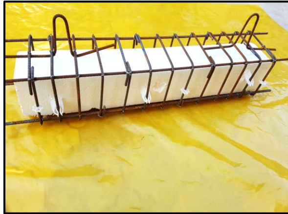
Plate 3.10: Compressed cork inside the reinforcement cage
