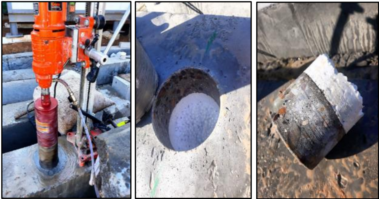
Plate 3. 1: Coring process
