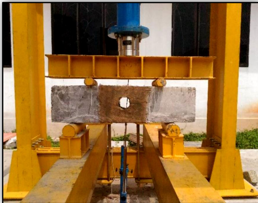
Plate 2. 5: Aramid fibre reinforced sheets wrapped around the opening of the tested beam used in the study of Garg et al. , (2017)
