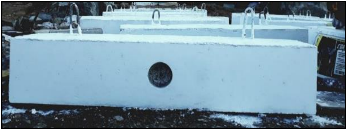
Plate 3.14: Beams after painting
