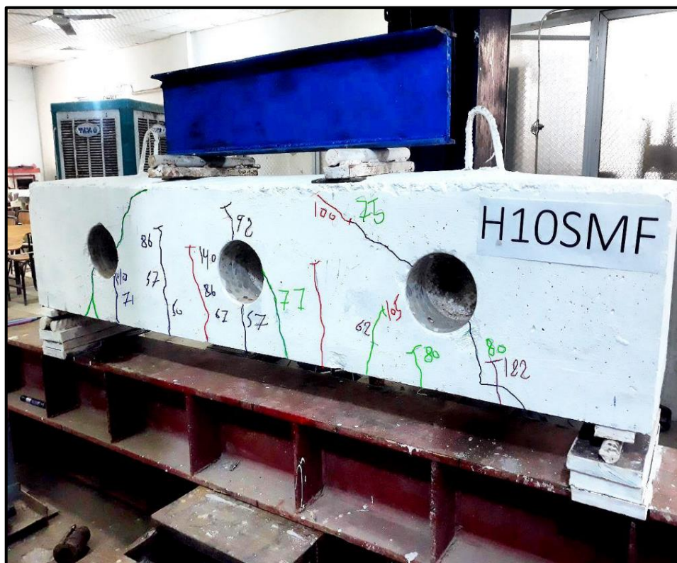
Plate 4. 4: Mode of failure and cracks pattern for (H10SMF)
