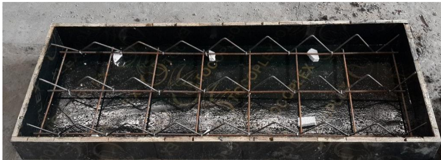
Plate (3-9): The Molds of Sandwich concrete slab.
