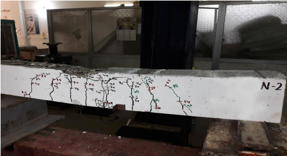
Plate 4-9: Cracks Patterns at Failure for N-2-28 beam specimen
