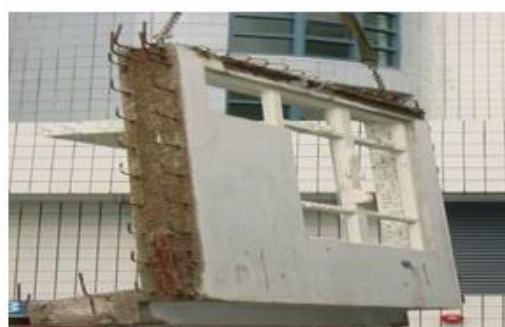
Protocol of finished lightweight concrete precast façade (25)
