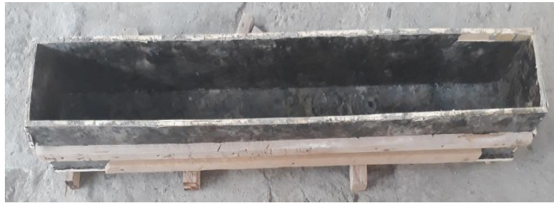
Plate 3-15: Plywood molds for beam
