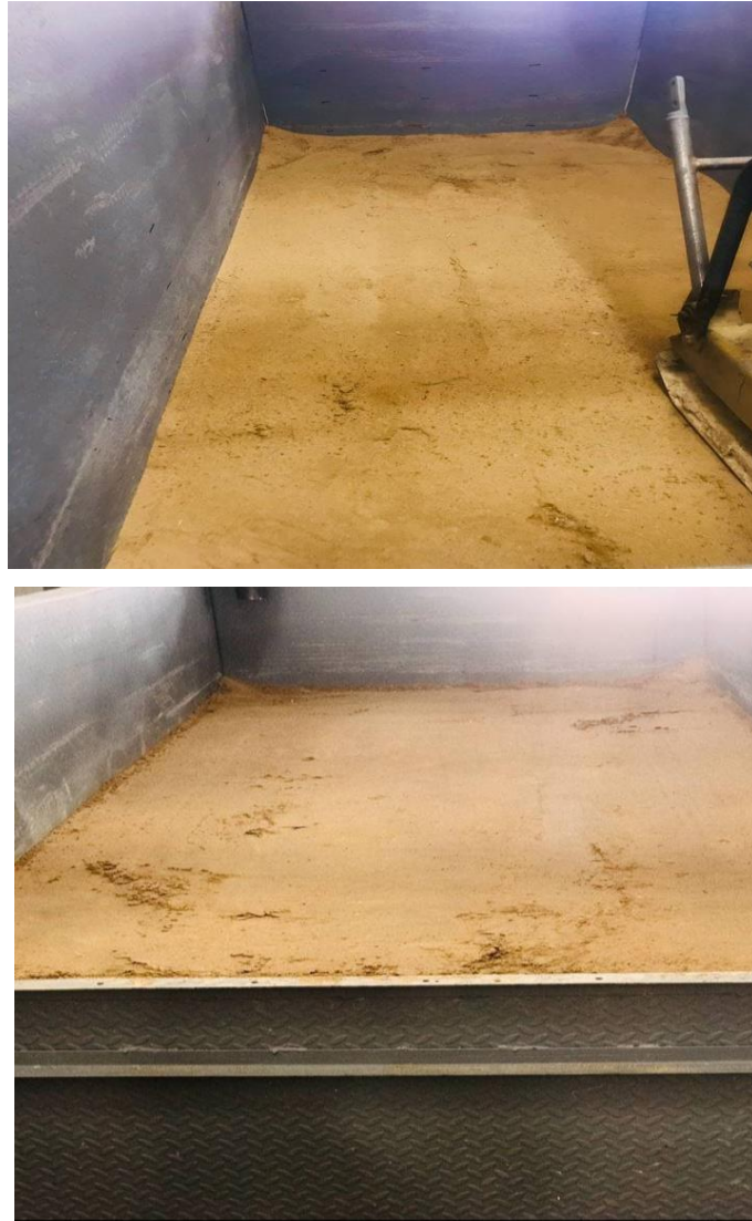
Figure 3-8: Illustrate Soil Preparation of Subgrade Soils.
