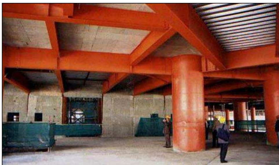
Plate (1.1) Composite steel storey system [3].
