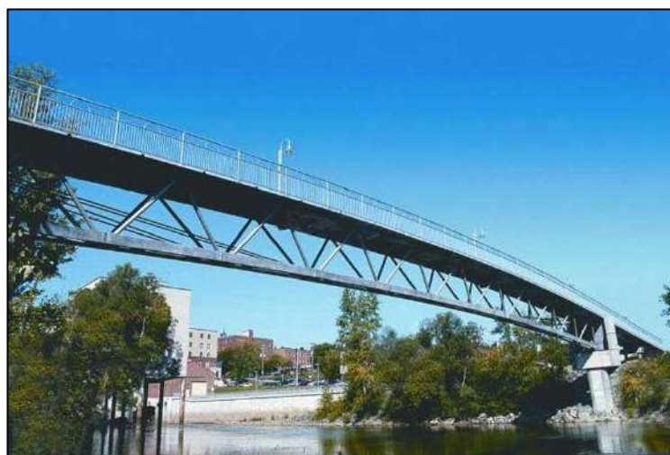
Plate (1.5) Sherbrooke footbridge [from google website]
