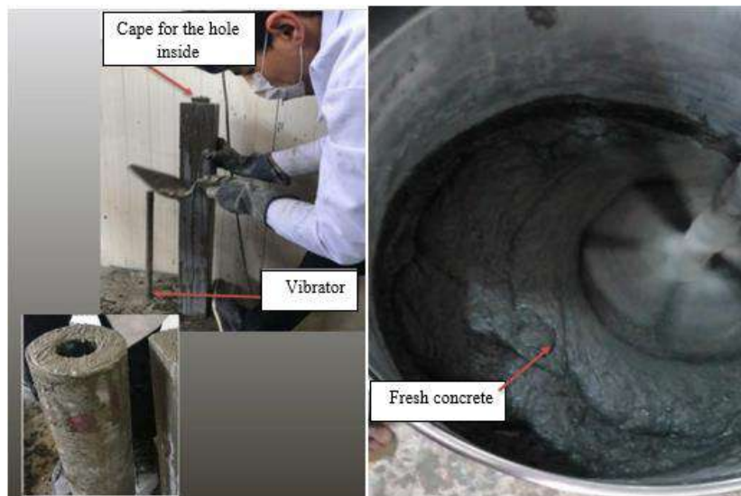
Plate (3.15) Mixing, placing and compacting of concrete.
