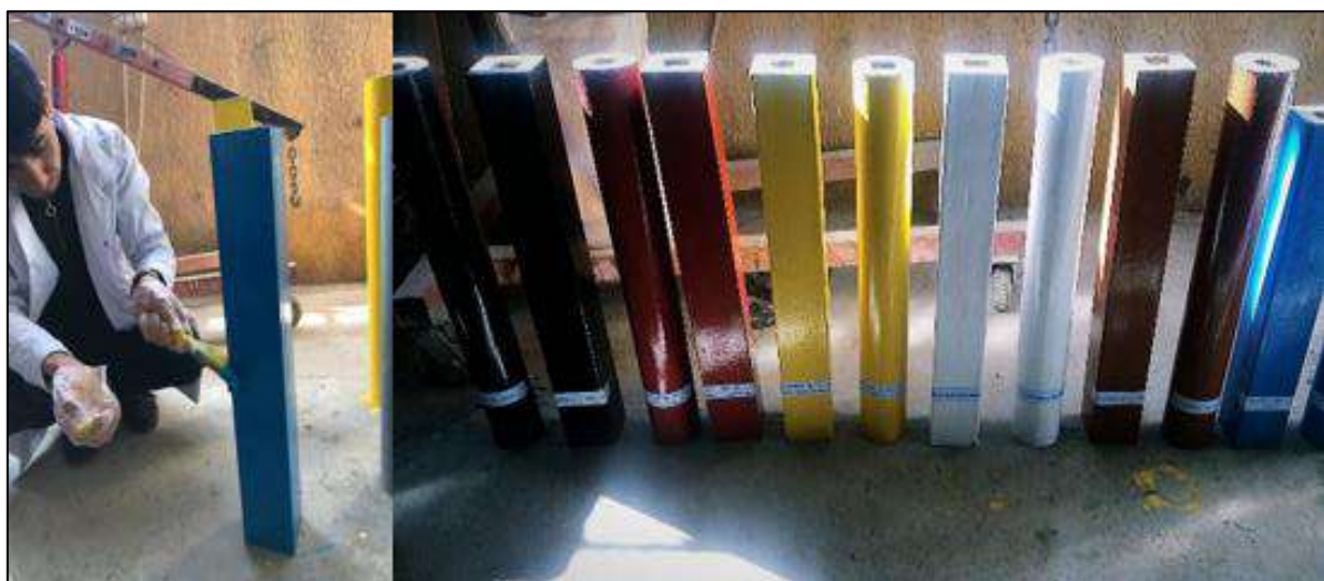
Plate (3.19)Coating of columns
