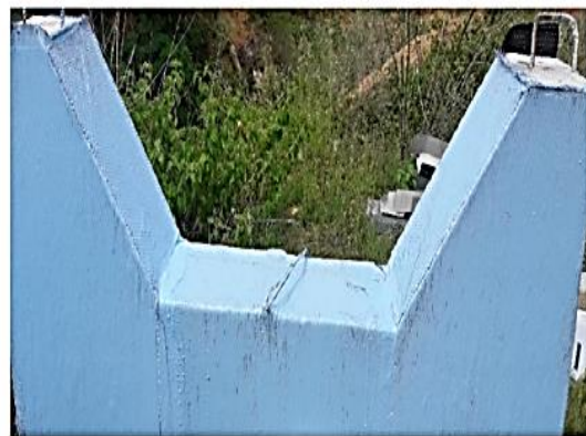
(iv) Finished Hybrid Repair specimen
