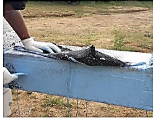
(ii) Grinding of Corners and Epoxy application
