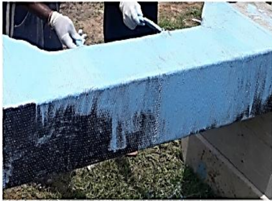
(iii) First Layer of FRP Wrapping
