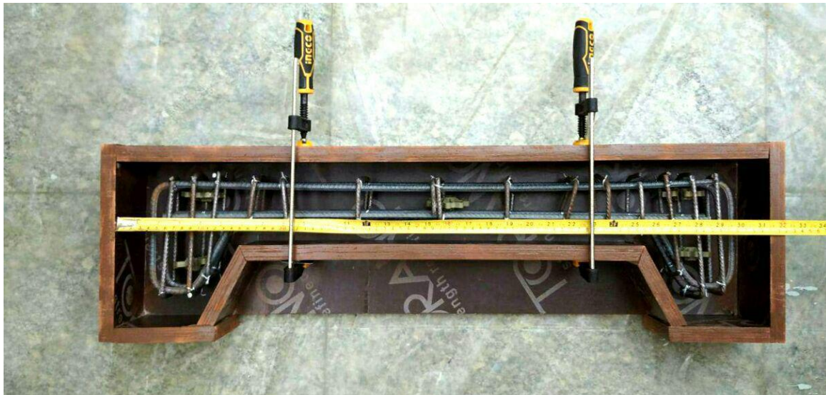
Plate 3. 4. Details of wooden mould for the column
