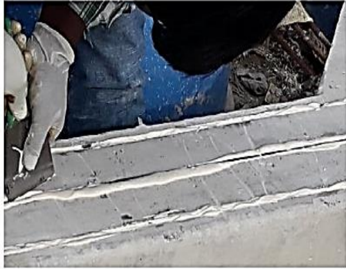
(i) Repair using NSM Technique
