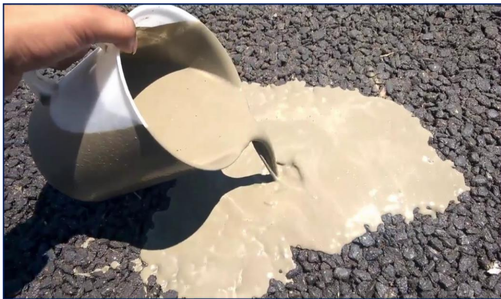
Plate (2-3): Formation of semi-flexible pavement
