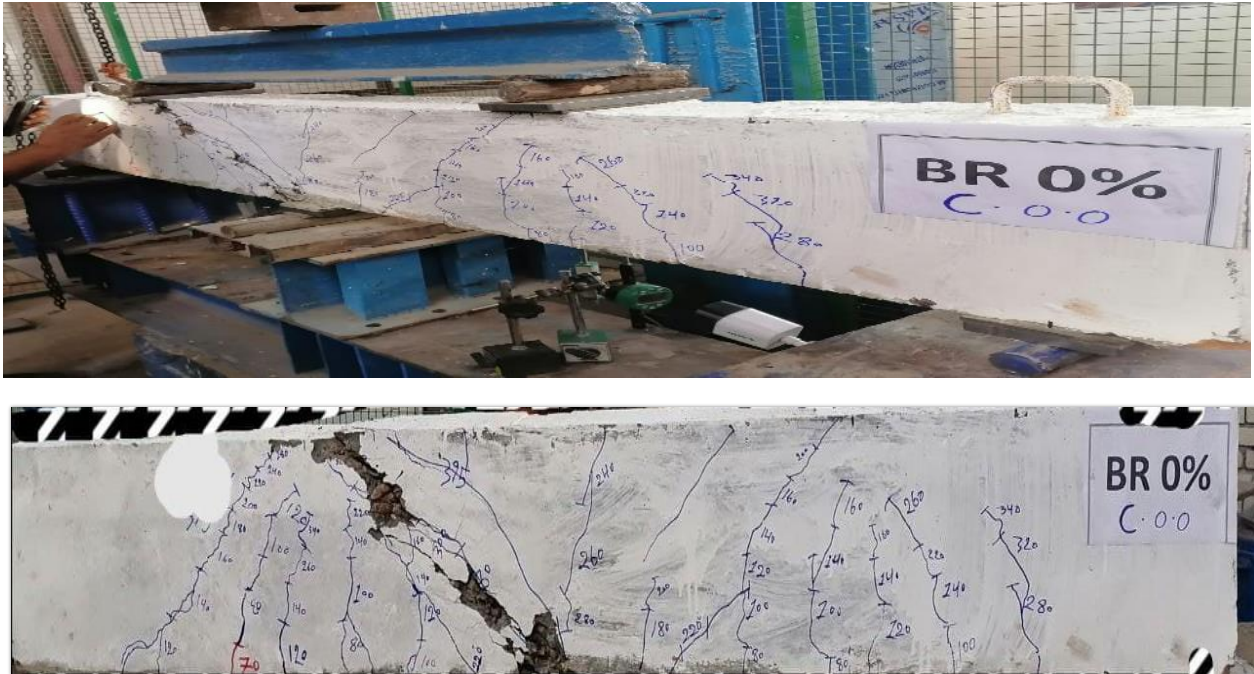
Plate 4.3 Cracks pattern for (BR0%) beam
