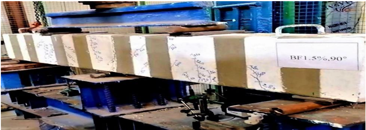
Plate 4.10 Cracks pattern after failure for (BF1.5%,90°) beam
