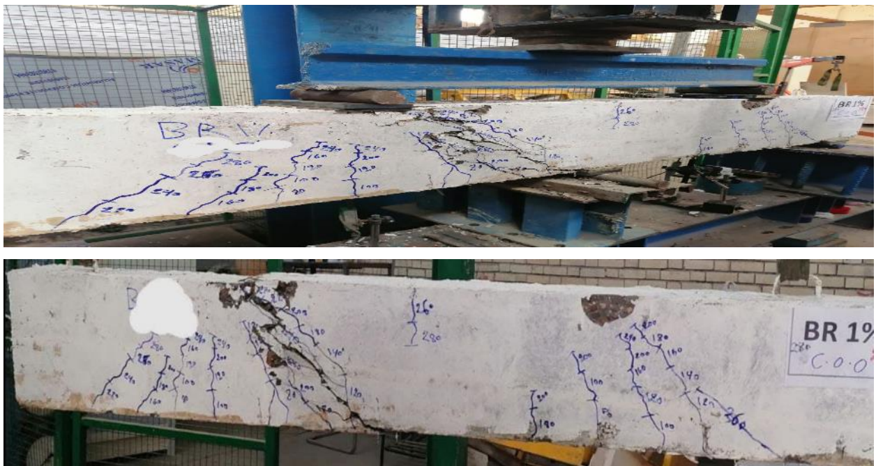
Plate 4.5 Cracks pattern for BR1%
