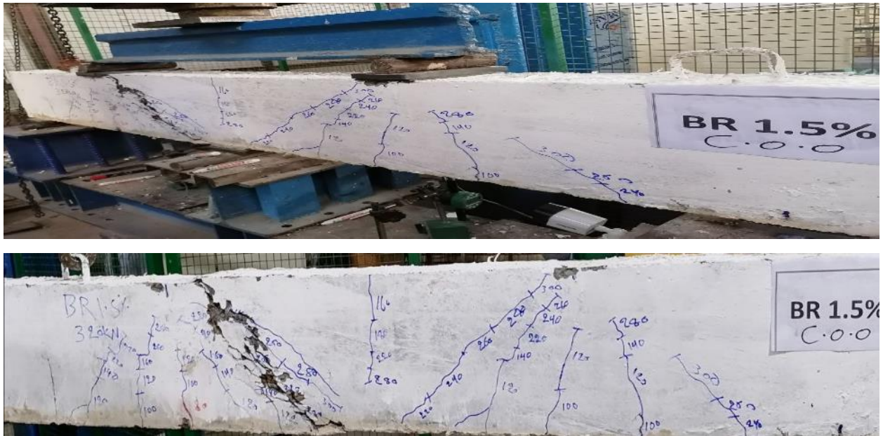
Plate 4.6 Cracks pattern for BR1.5%
