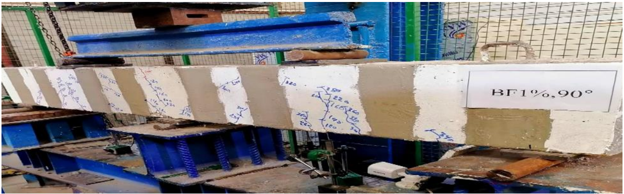
Plate 4.9 Cracks pattern after failure for (BF1%,90°) beam
