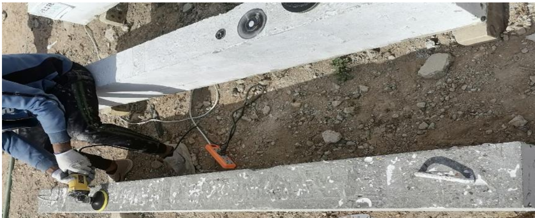
Plate 3-8 Removing the painting from the beam surface
