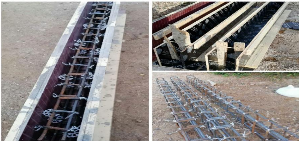
Plate 3-6 Plywood formwork and reinforcement of specimens
