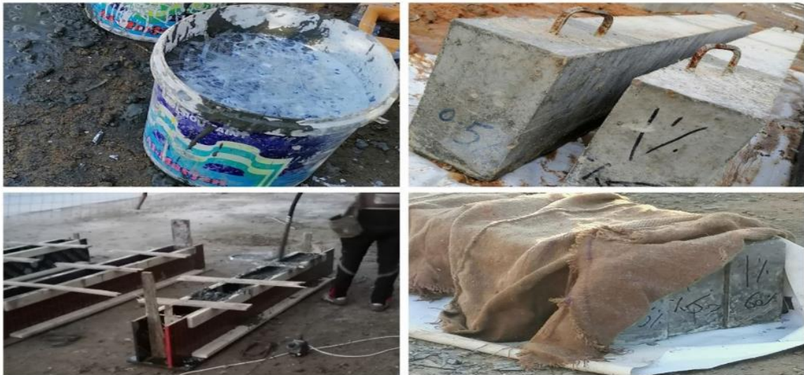
Plate 3-7 Casting and Curing Process
