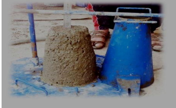
Plate 3-3: Slump flow for fresh concrete test
