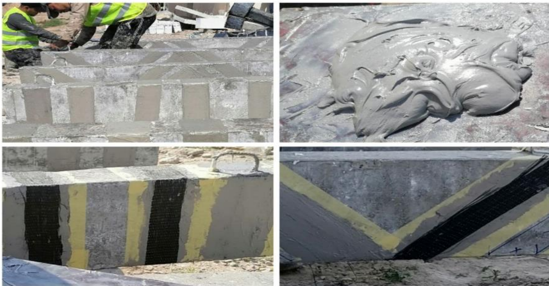
Plate 3- 9 Steps of CFRP Fixing
