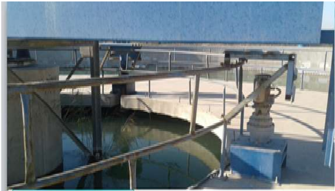
Plate (1-1): The appearance of plants inside the sedimentation basin at the water treatment plant in Kerbala.
