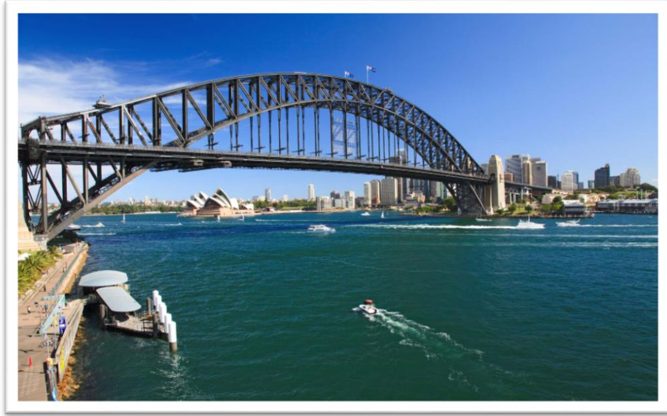
Plate (1.3): Sydney Harbour Bridge (Image Source: https://www.britannica.com/topic/Sydney-Harbour-Bridge )
