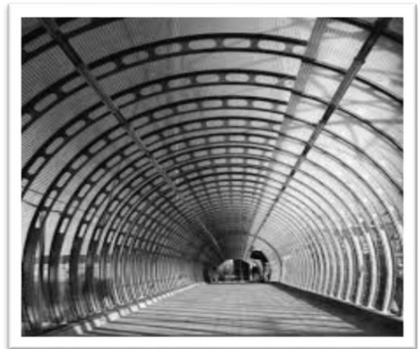
Plate (1.2): Arched Steel Beams in Walkway [5]
