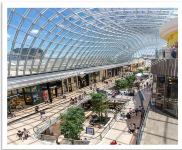
Plate (1.1): Arched Steel Beams in Roof of Retail Centre (image source: https://seele.com/references/chadstone-shopping-centre )
