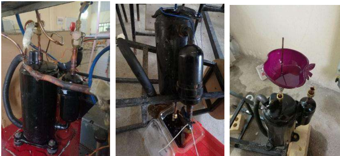
Figure (4.9): Process of charging the lubricant oil.
