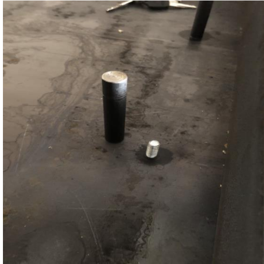
Figure 3-7 steel shafts installation process
