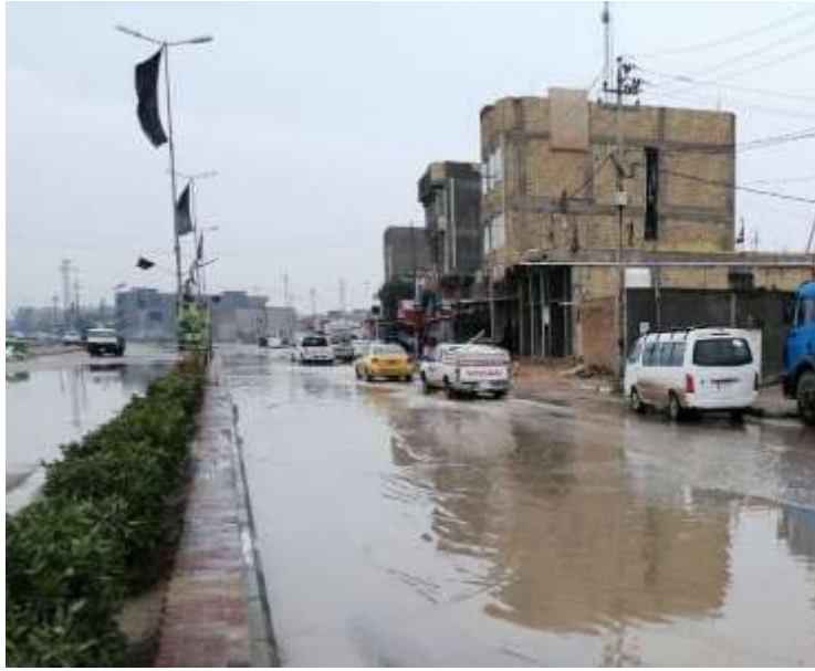
Figure A-3: Flooded area in Al-soob Al-Kabeer Quarter (picture taken in Feb. 2021)
