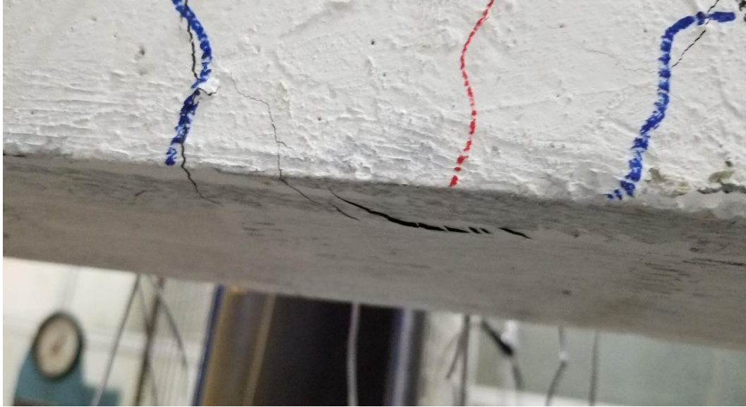
b): The peeling stress is spread over a wider area under the surface beam
