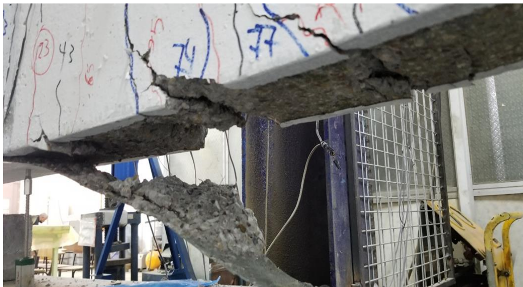
a): Crack Patterns and Failure Modes
