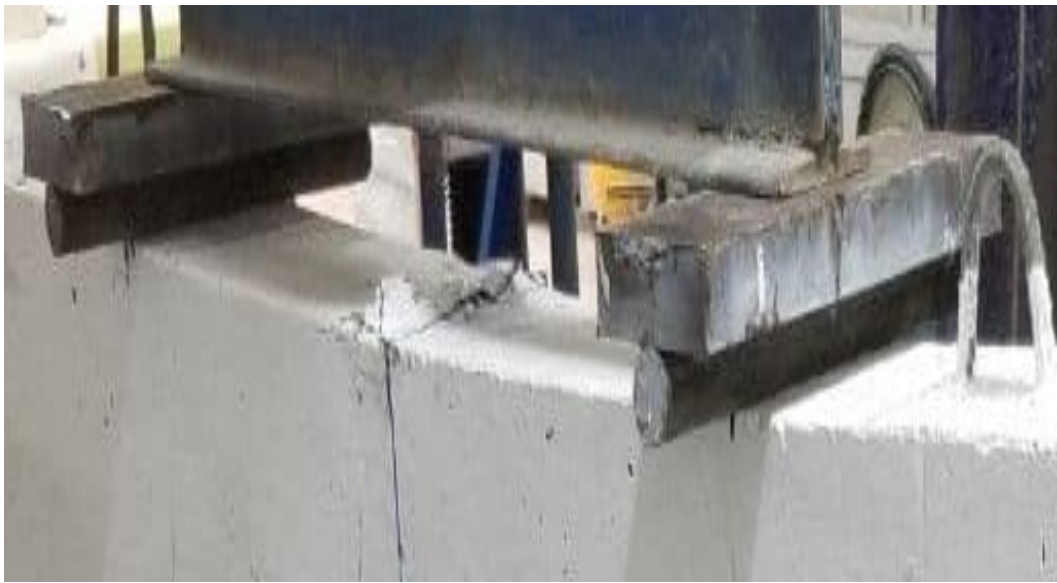
c): Final loading stage, additional cracks developed from the top surface in the middle of the beam
