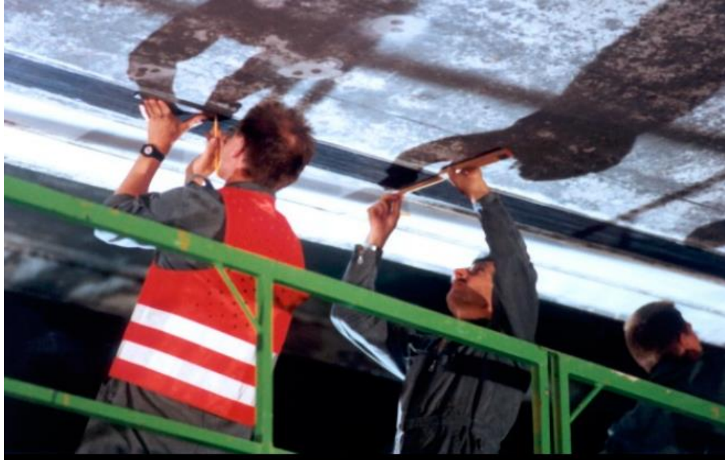
Figure 2-6: Strengthening work on the Ibach bridge in the year 1991.
