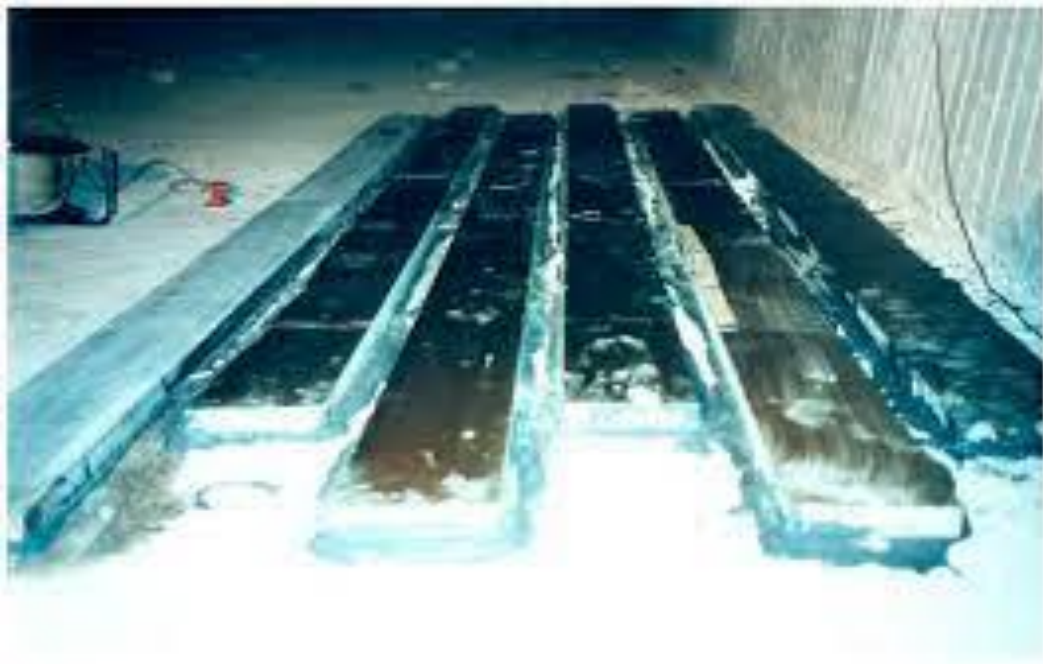
Figure 2-4: Glass fiber reinforced polymer (GFRP) Plates at the bottom slab of Kattenbusch Bridge.[43]
