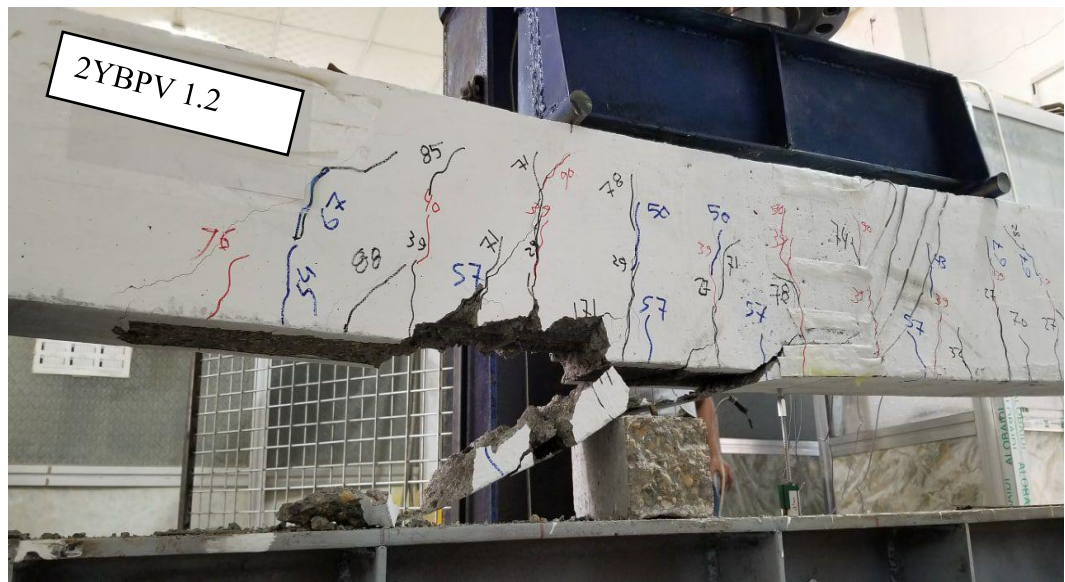
b) The failure of the beam by cover delamination
