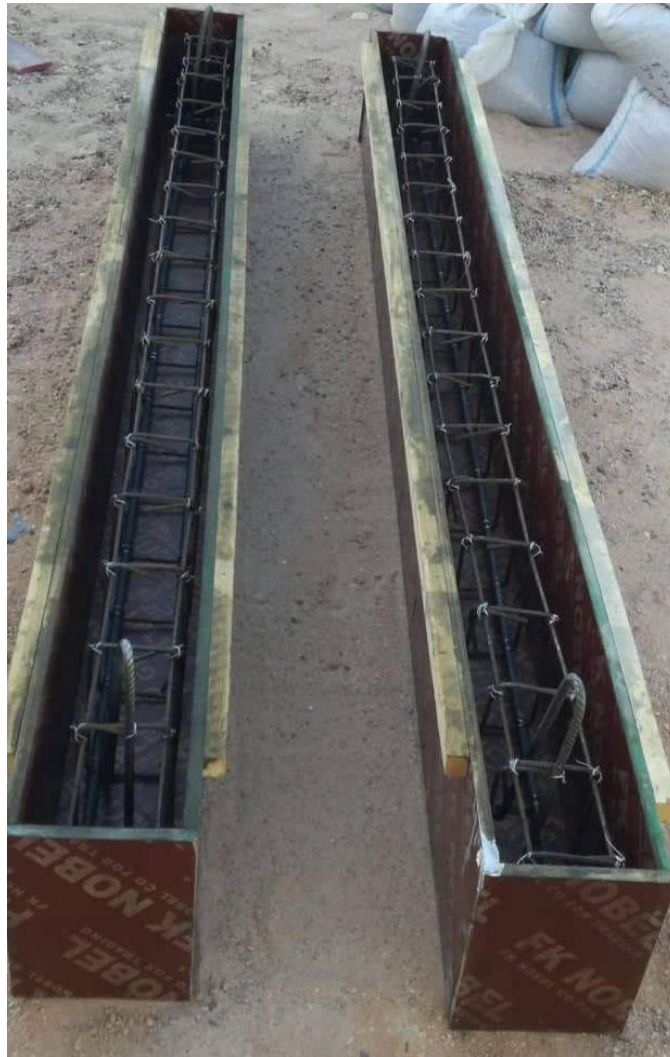
Figure 3-11: The plywood formwork with the reinforcement.
