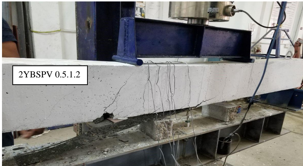
d) Failure of the beam 2YBSPV 0.5.1.2 by debonding problem
