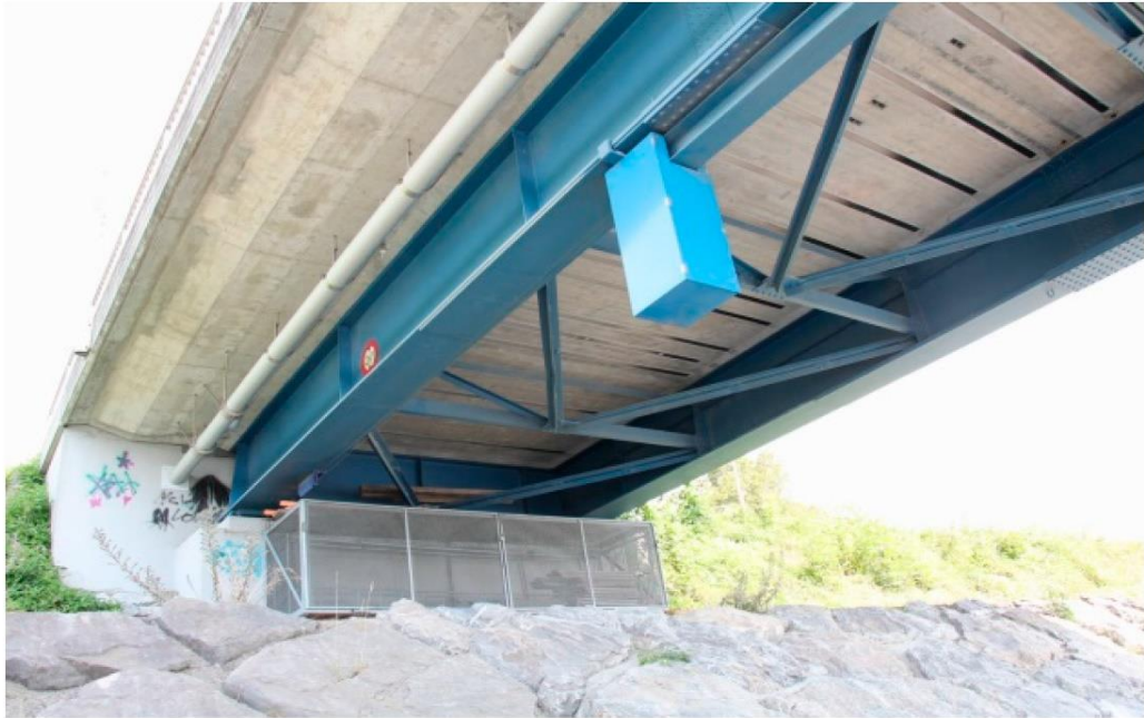
Figure 2-7: Bridge over the river Rhine near Oberriet in Switzerland
