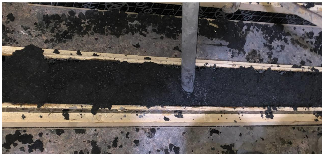
Plate 3-11: Beam specimens cast.
