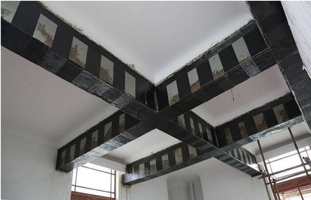
Plate 1.3: The application of CFRP in the strengthening of beams [ Khan, 2002 ].
