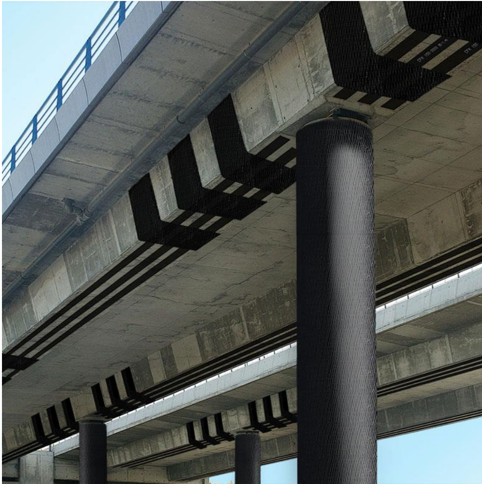
Plate 1.1: Overview of the FRP strengthening work [Klaiber et al., 2003].
