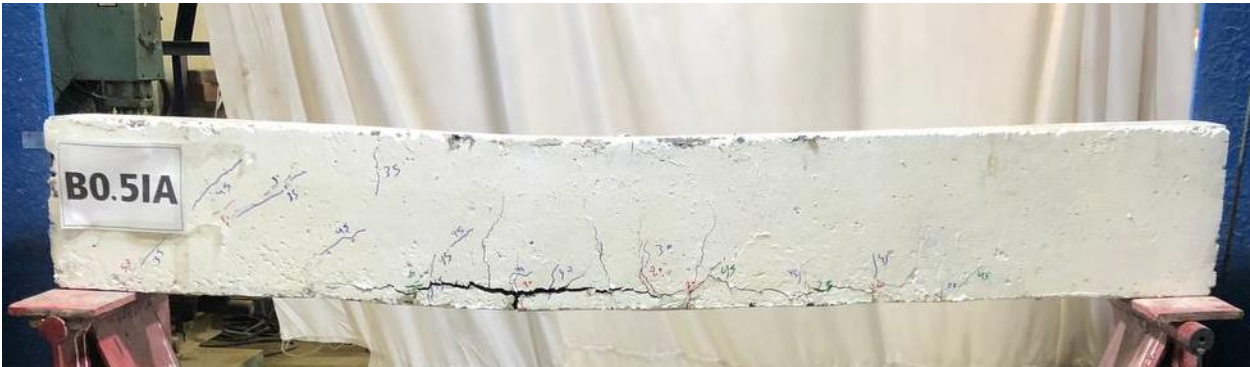
Plate 4.8: Cracks Pattern of Specimen B0.5IA.
