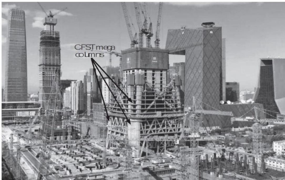
Figure 1-5: Shows the use of CFST in the construction of tall buildings in China (Han, Lam, et al., 2018)
