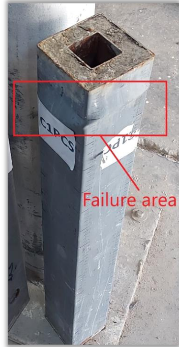
Figure 4-2: C1PCS Column failure
