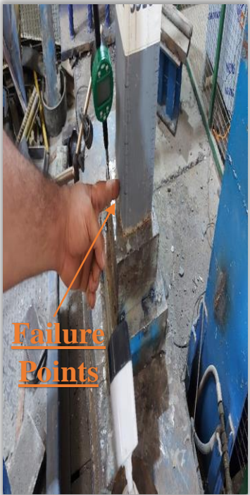
Figure 4-26: C2FCS column failure
