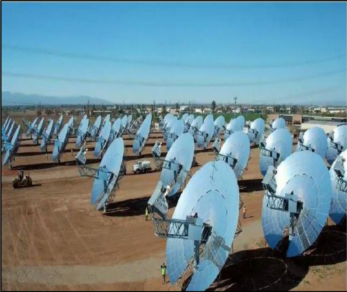
Figure (1.3): Parabolic Dishes (DP) [6]
