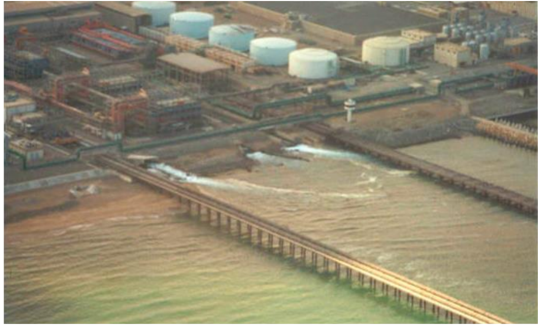
Figure 2.7 : Surface discharge of the Al-Ghubrah desalination plant, the largest such facility in Oman
