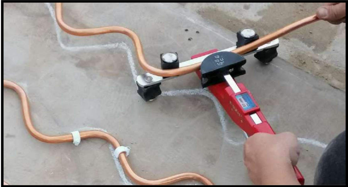
Figure 4-4: Wavy Shape Pipe Manufacturing.
