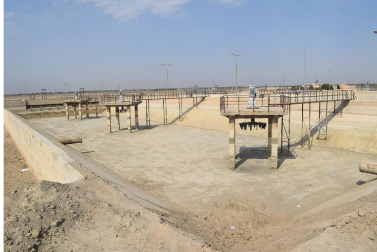
Figure 3-6. Aeration Basins in WWTP of AL-Samawah taken by Zahraa on October 28 th , 2021).
