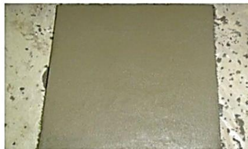
(h) Finished strengthened slab
