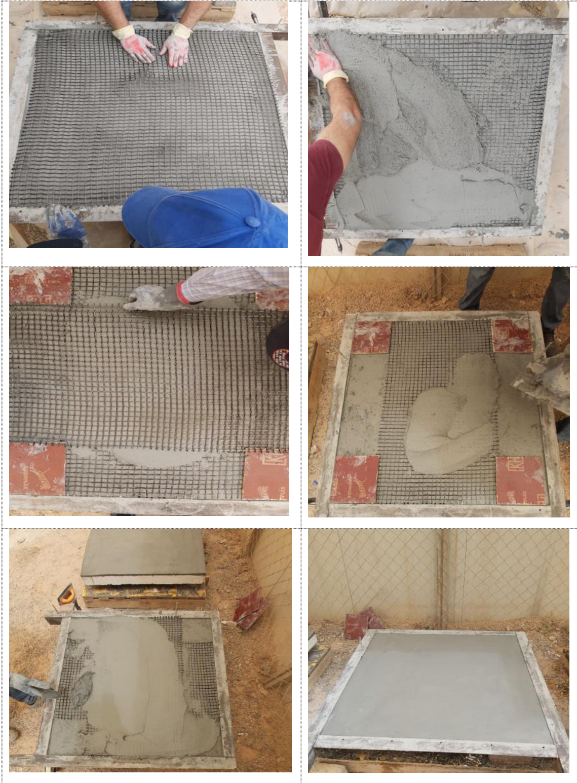
Figure B-5: TRM layers application steps.
