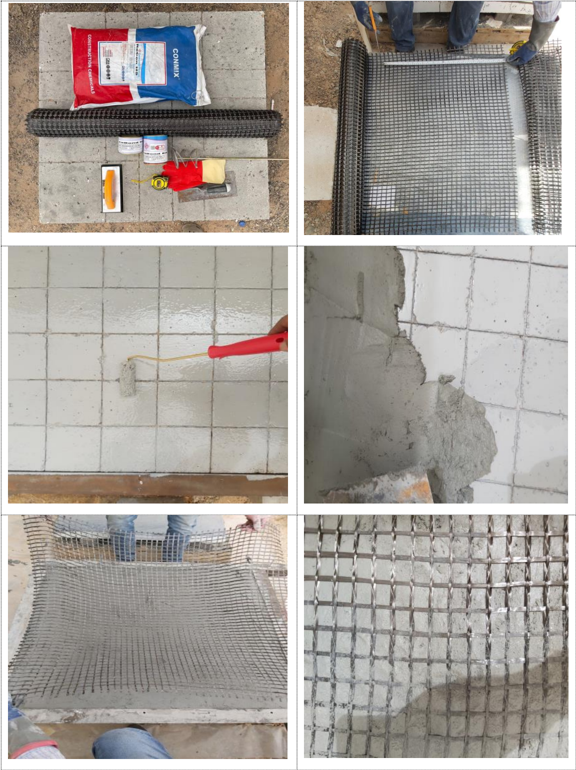
Figure B-4: Steps of application TRM layers.
