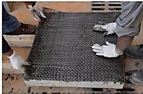
(e) Pressing on fabric for mortar penetration
