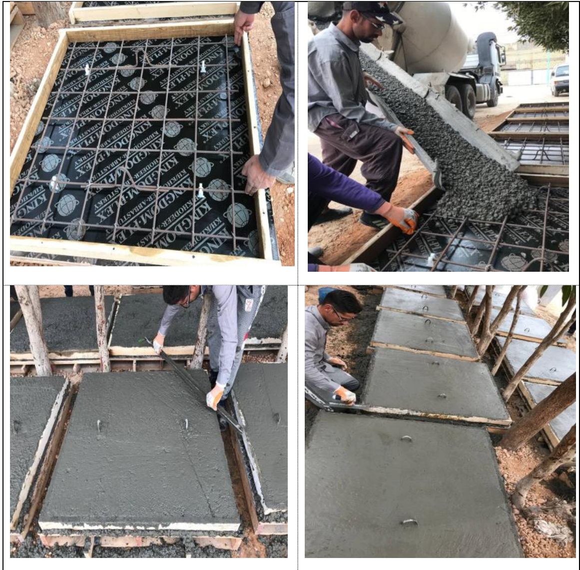
Figure 3-6: Steps for pouring concrete slabs.
