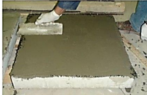
(f) Saturation of I layer of fabric with mortar
