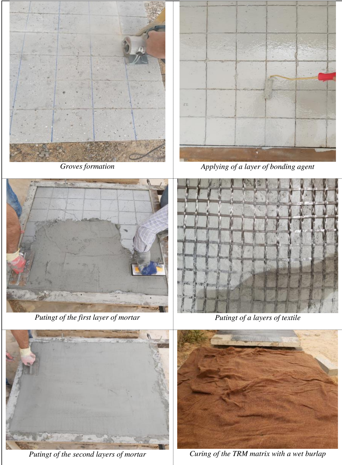
Figure 3-15: Application of TRM layers at the tensile face of tested slabs.
