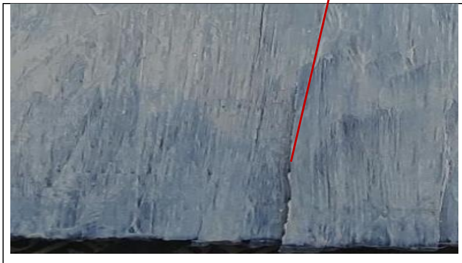
Figure 4-5: Rupture of a Small portion of CFRP fibers near the supporters in the tension zone (S4).
