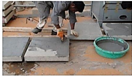
(b) Sika Armatec Epo cem application as bonding agent
