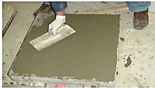
(c) First layer of Sika Rep mortar application
