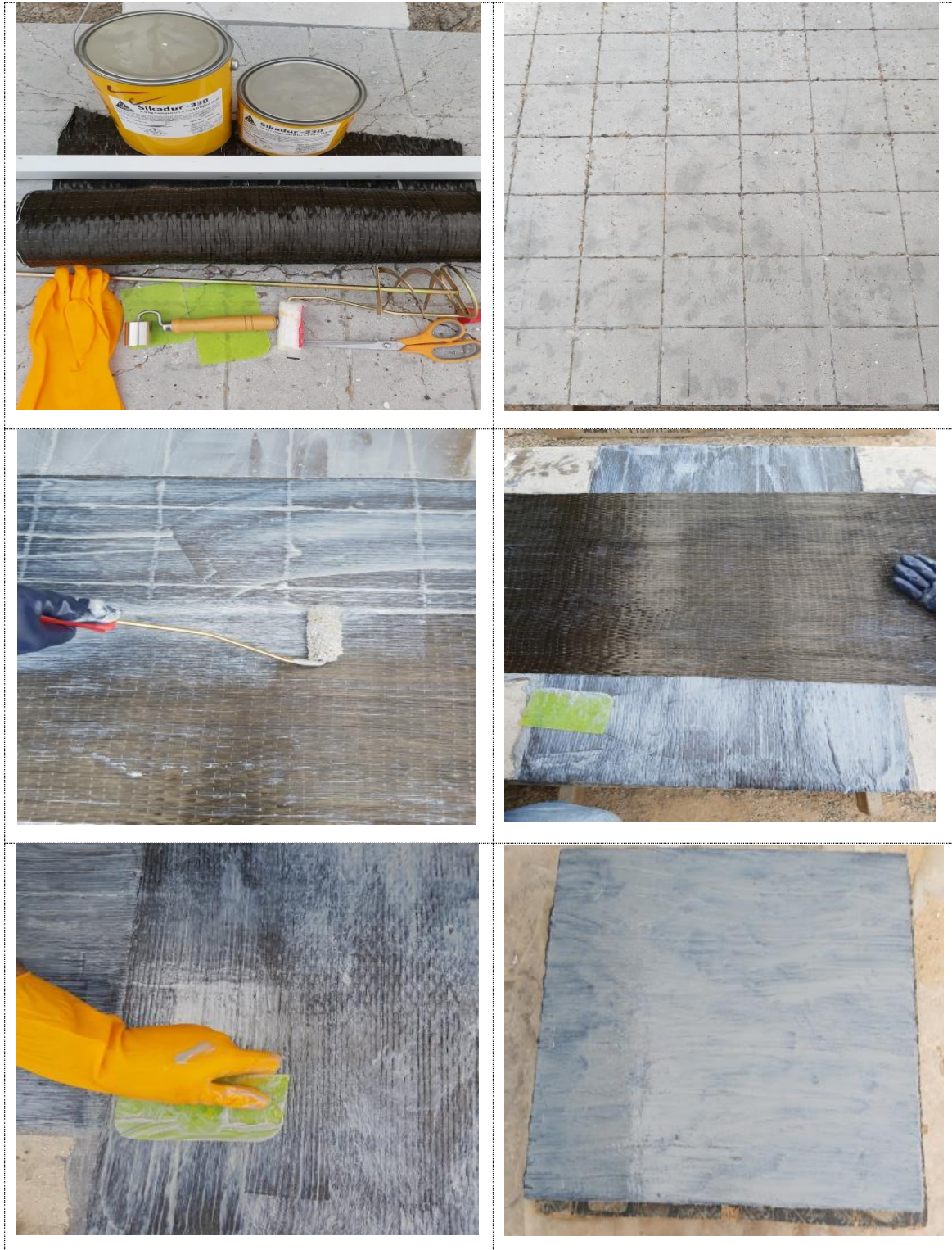
Figure B-2: Steps of application CFRP sheets.
