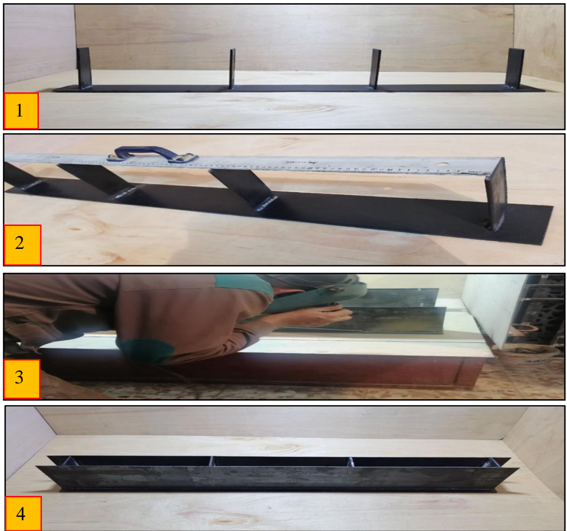
Figure 3-6: Steps Welding Process of Double Web Beams.
