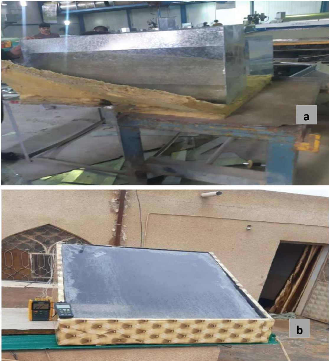
Figure (4.1) The solar still collector components (a)Manufacturing a solar still (b)Installing the device on the rooftop
