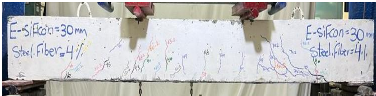
Figure 4.16: Cracking Pattern of Specimen E30-4F.
