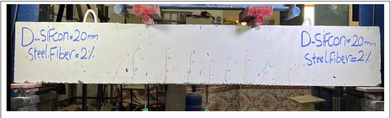
Figure 4.12: Cracking Pattern of Specimen D20-2F.
