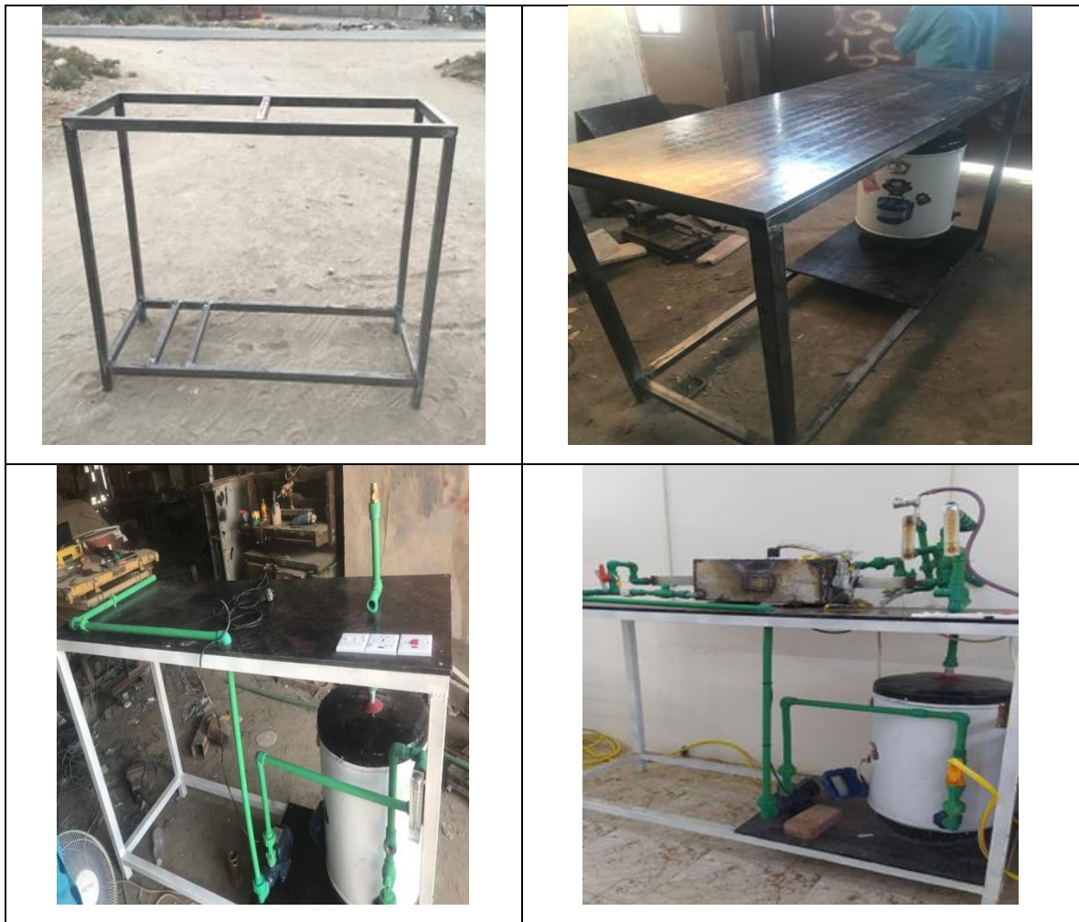
Figure 4.7: Preparing the water source and connecting it to the pump, heater and TSCTSU
