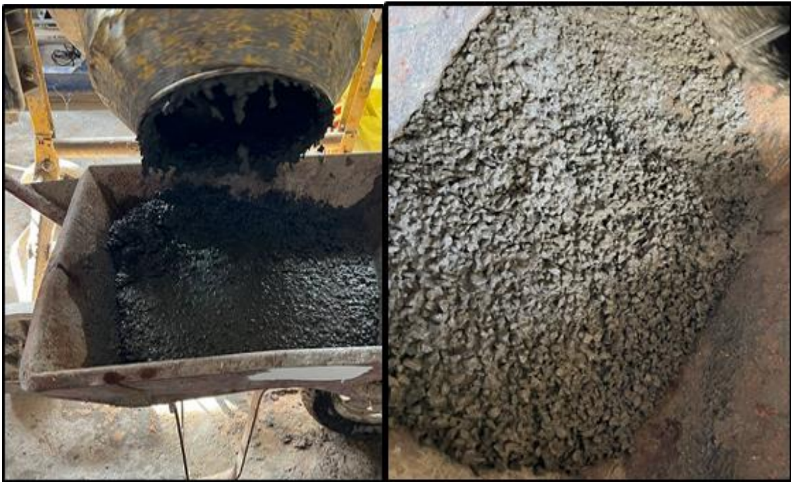
ate 3-17 Mechanical Machine Supply Normal Concrete (NC)
