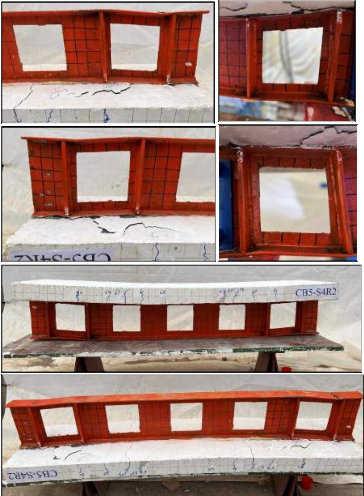
Plate 4-36: Beam CB-S4R2 at Failure.
