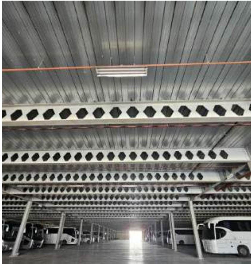
Plate 1-1:Some Uses of Castellated Steel Beams (Alkafeel Garage).
