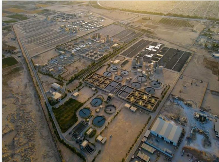
Figure 3-1. Google Earth Satellite View of the Karbala WWTP.
