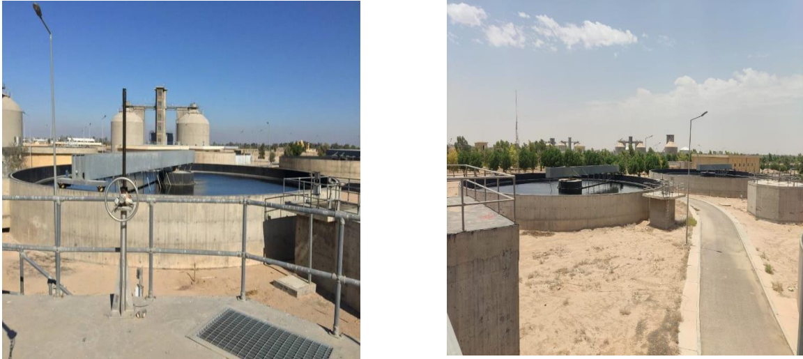
Figure 3-7. Secondary clarifier tank of Karbala WWTP.
