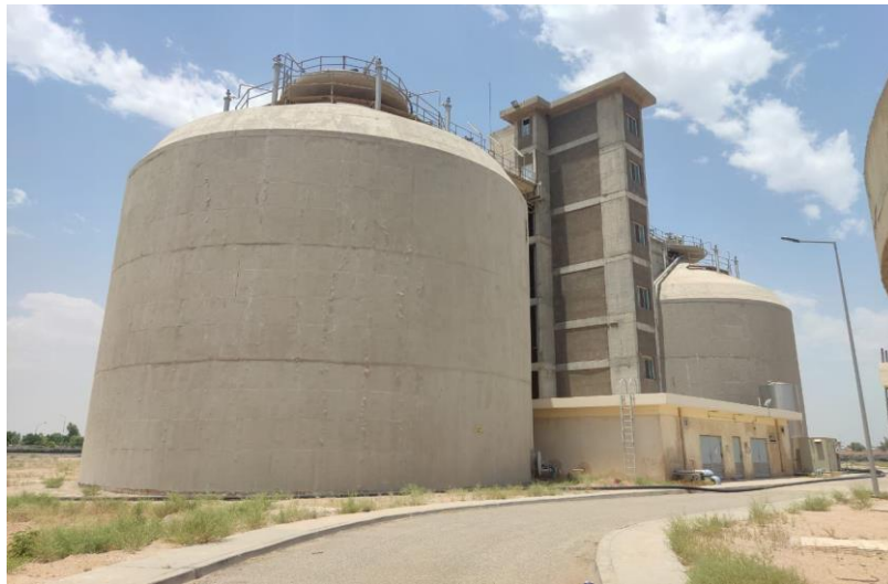
Figure 3-10. Anaerobic digester of Karbala WWTP.
