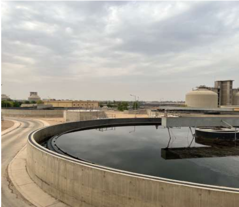
Figure 3-7: Secondary Clarifier Tanks of Karbala WWTP
