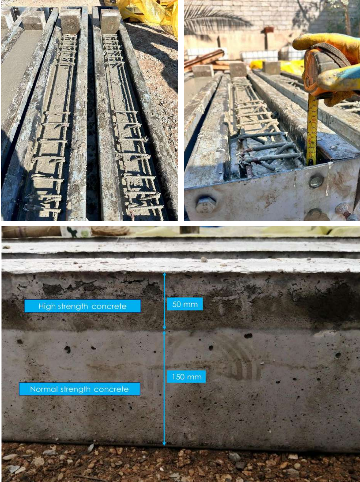
Figure (3.17): Formwork and casting of the bilayer concrete.
