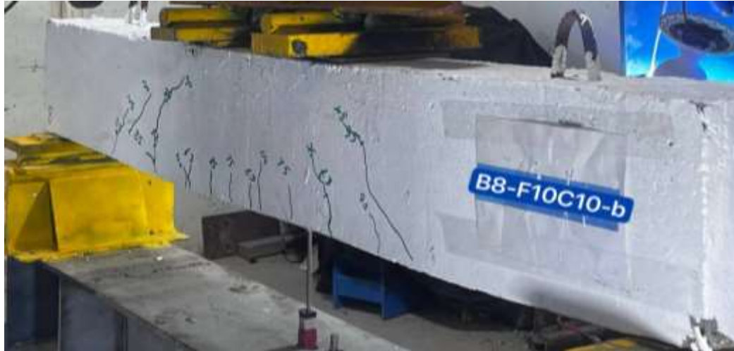
Plate 4-10: Failure mode for B8-F10C10-b under repeated load
