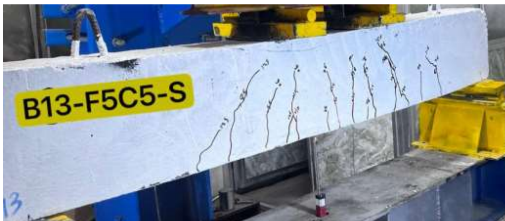
Plate 4-15: Failure mode for B13-F5C5-S under repeated load
