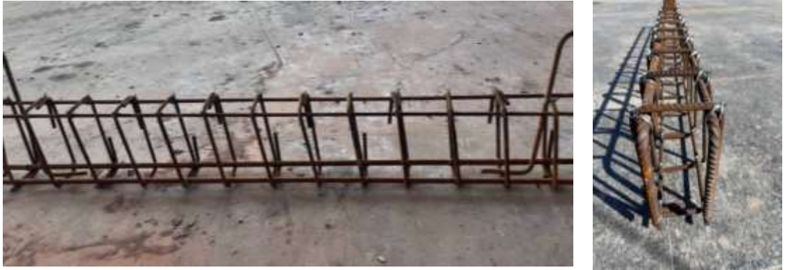
Plate 3-2: Steel reinforcement details.
