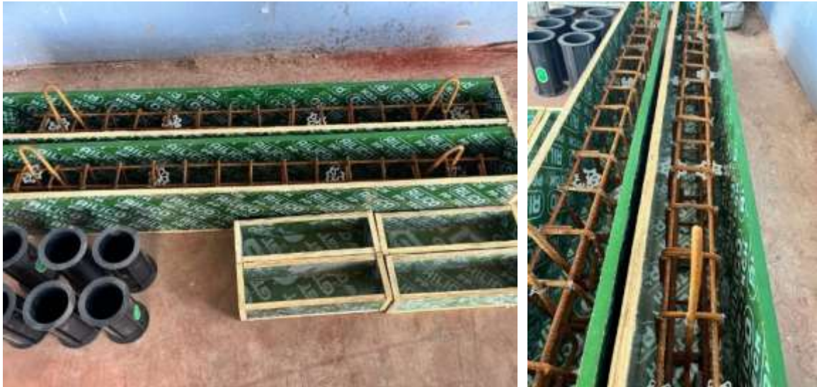
Plate 3-8: Preparation of plywood formwork and reinforcement
