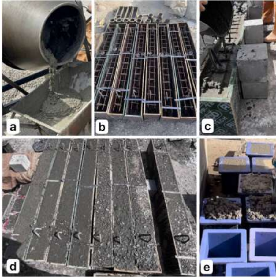
Plate 3-9: (a) Casting of concrete ,(b) Preparing the molds ,(c) Pouring concrete mix into molds (d) The shape of the molds after casting,(e) Cube modeling.
