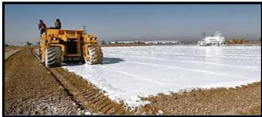
Figure (2-2): Application of Lime Stabilization(Mr. Mukherjee , 2014).
