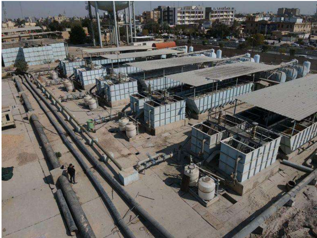
Figure (3-2): Al-Hussein Neighborhood Water Project ( Al-Hussein neighborhood water project, 2023 ).
